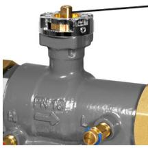
A Rotating the stem of the control valve (A) will modify the  $K_v$  of the valve, thereby altering the flow rate.
